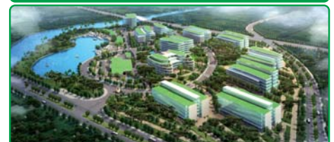
BSD City Green Office Park, Indonesia
